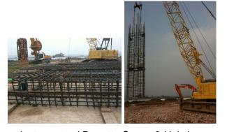
Instrumented Barrette Cages & Hoisting Testing was successfully completed with a load of approximately 32.0 MN applied to each test.
