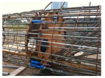
O-cell Assembly in Pile Cage (Bored Pile)
